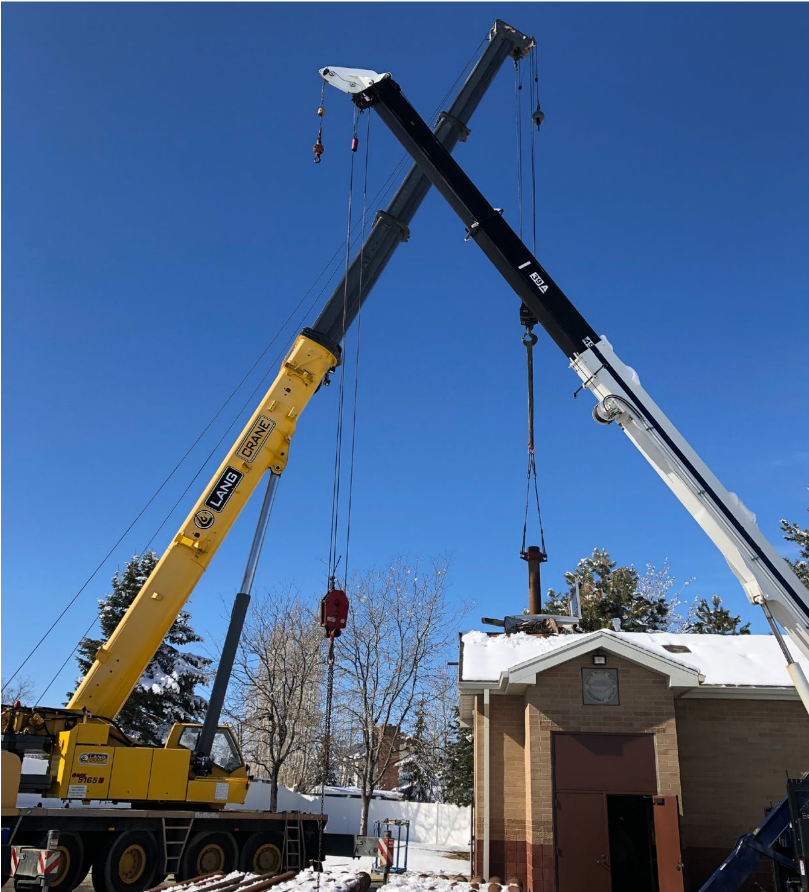
Removing pump equipment at Newbury Well
