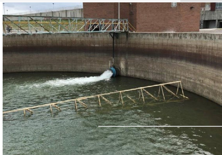
JWTP Backwash Clarifier Start-up Testing - D. Martin
