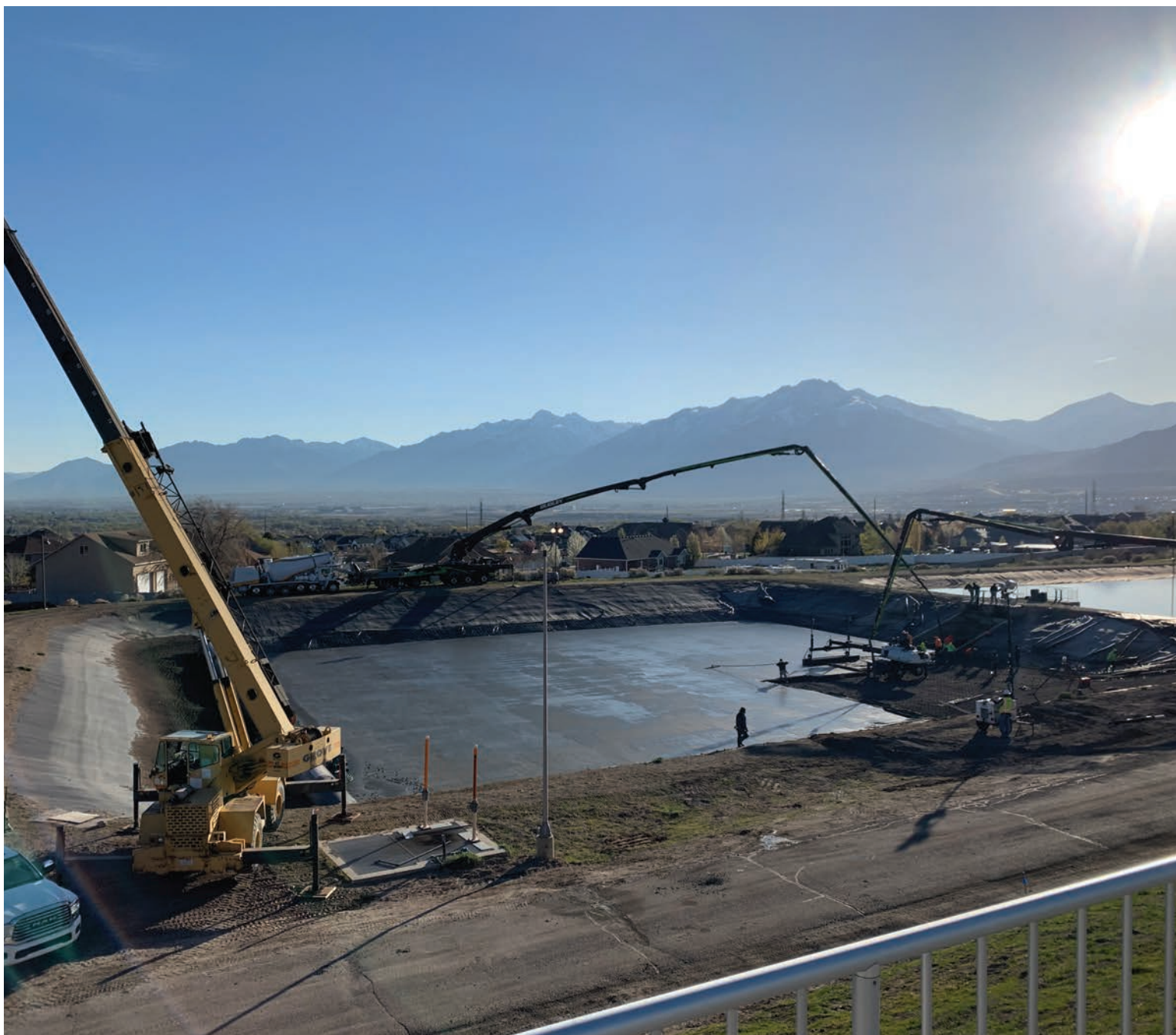
Pouring concrete bottom in the JWVTP backwash lagoons - A. Kimmerle
