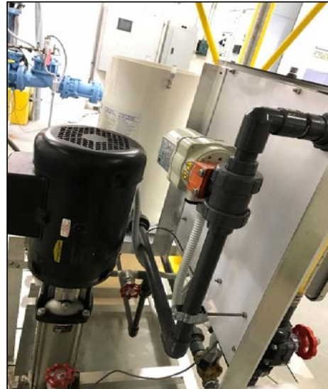
Typical analog valve providing remote chlorine setpoint control
