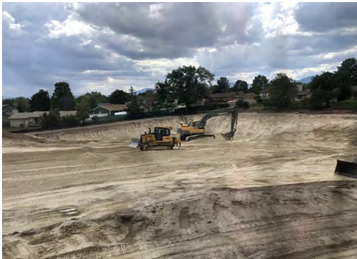
Excavation of the new reservoir site
