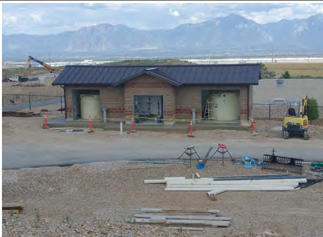
The chemical feed building with sidewalk, roof, and chemical tanks installed
