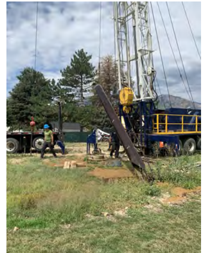
Bailing material from the well
