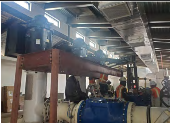
Installation of the platforms around the pumps and motors
