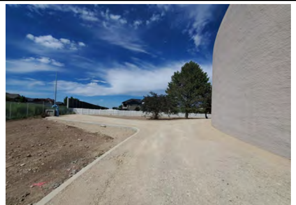
New roadbase maintenance road around the reservoir
