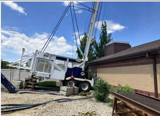
DW7 During Well Development
