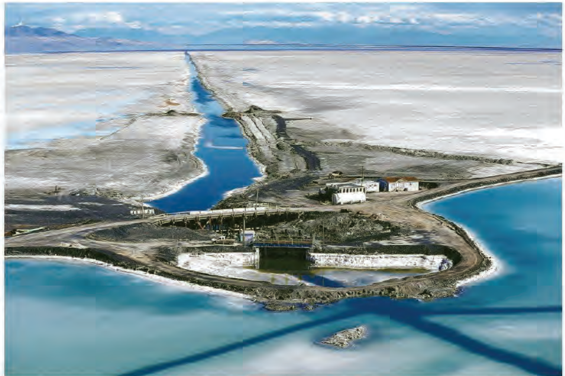
The west end of the Behrens Trench of Compass Minerals is seen on Oct. 18, 2016. The trench moves brine from the west pond complex to the east pond complex of Compass Minerals. Ravell Call, Deseret News
