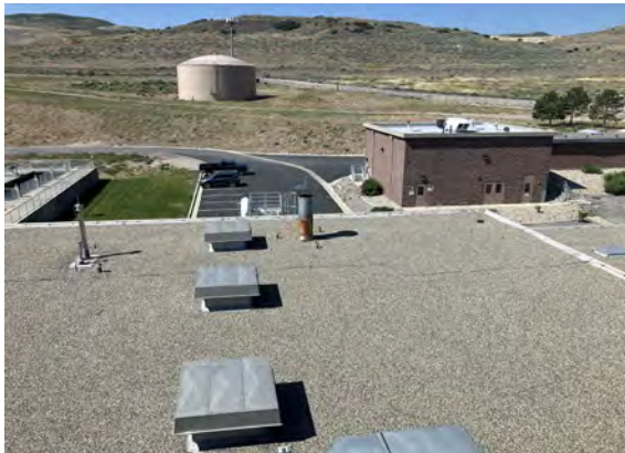
Existing JWTP Backwash Tank
