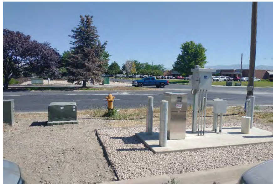
Finished construction with new transformer, pad, power meter, rectifier, and cathodic well
