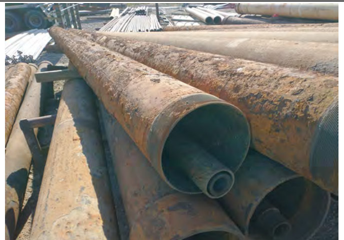
Corroded shaft and column
