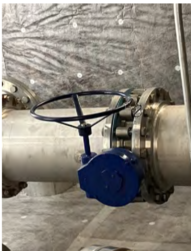
Installed acoustical insulation
