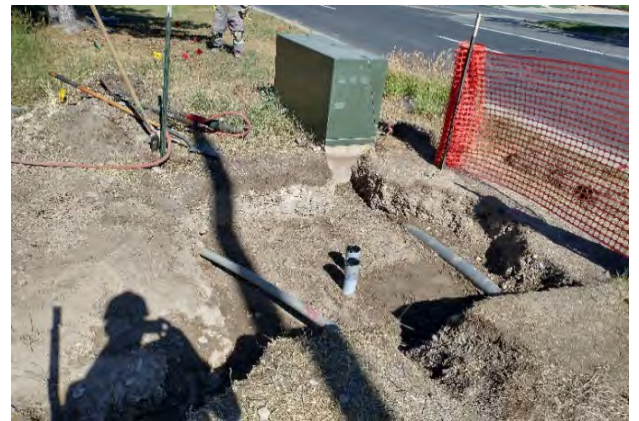
Excavated pit for new power transformer
