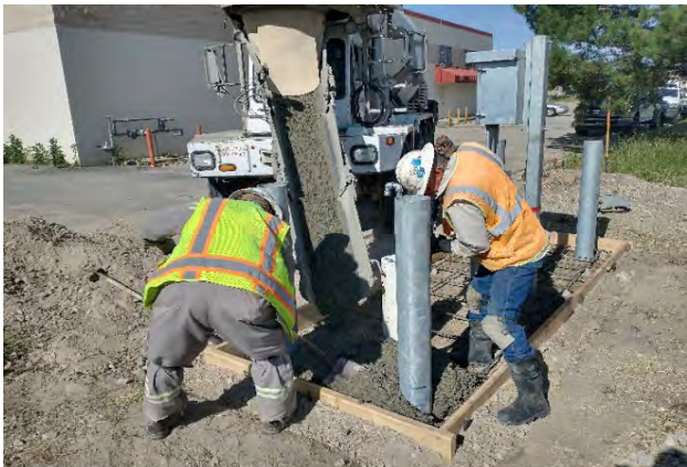
Pouring new concrete base for well, rectifier, and meter pedestal
