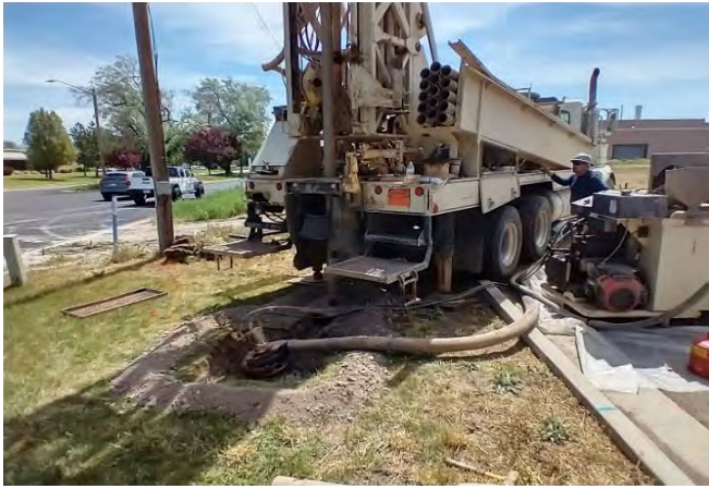
Drill rig drilling cathodic well
