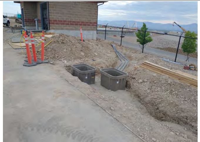
Installing buried electrical conduits and electrical pull boxes
