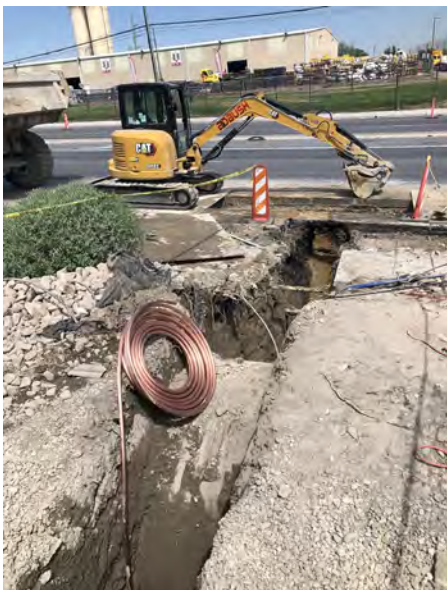
Installing ¾" service lateral
