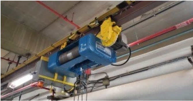
New crane hoist (blue)
