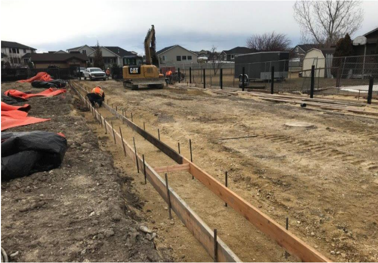
Construction of new entrance road.
