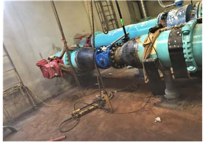
Construction work in progress
