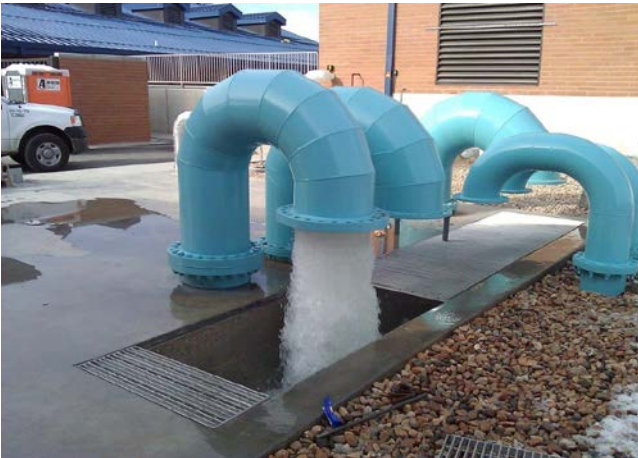
Aqueduct drain in progress using upgrades of this project
