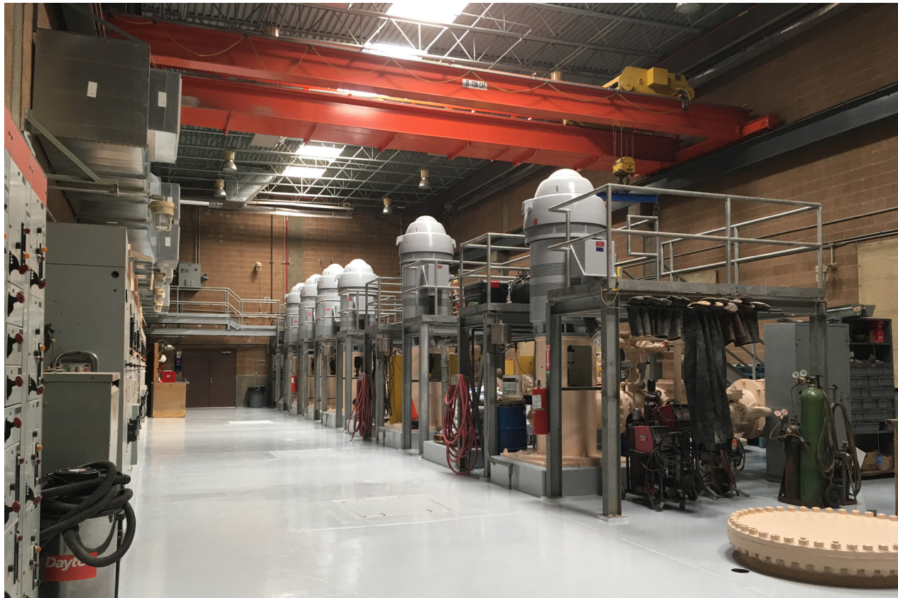
Above: Willow Creek Well Pump Replacement.
