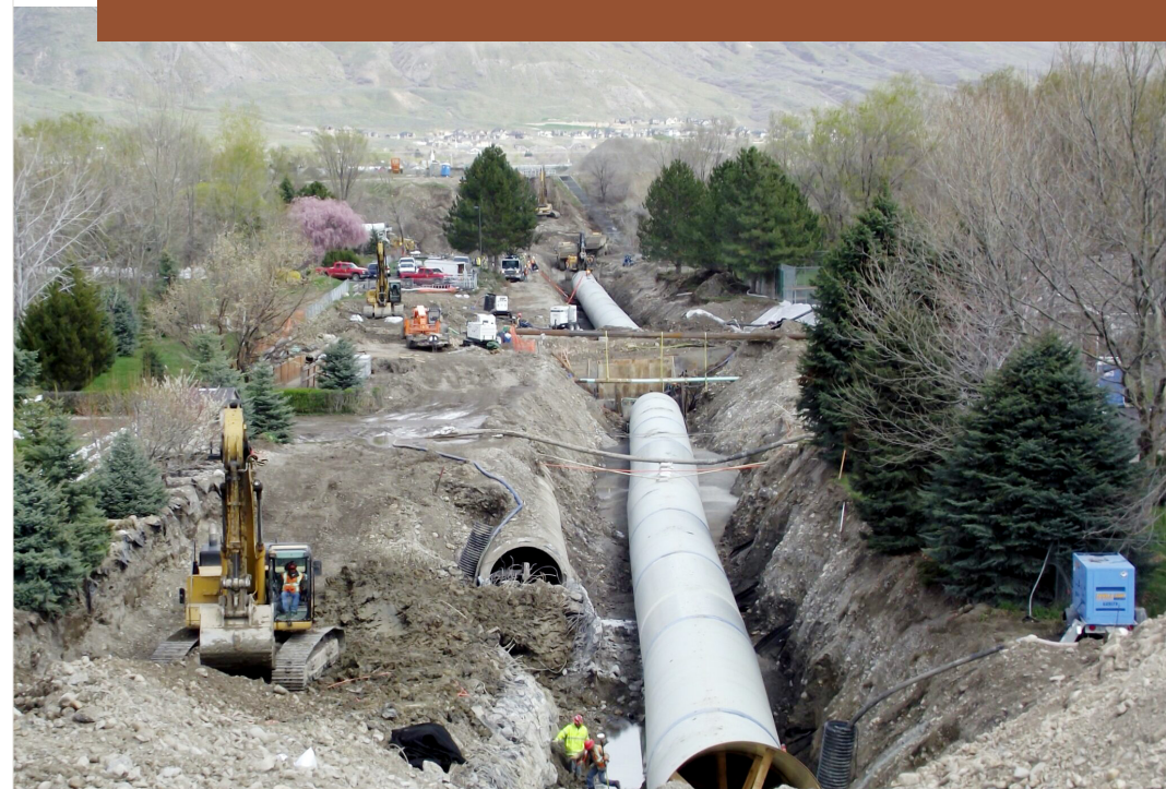
Installation of the Jordan Aqueduct
