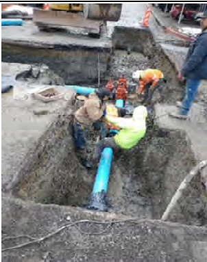
Installing a new 3-valve connection at intersection
