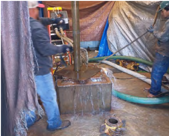
Retrieving the dual swab tool from the well
