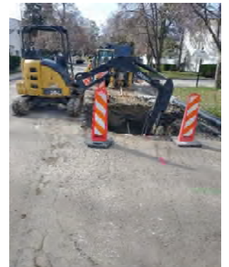
Directional drilling tool drilling hole under creek
