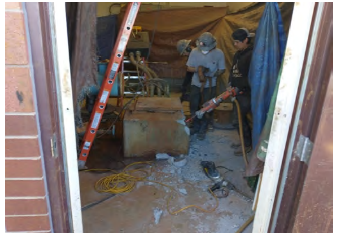
Jackhammering into floor to uncover gravel feed tube
