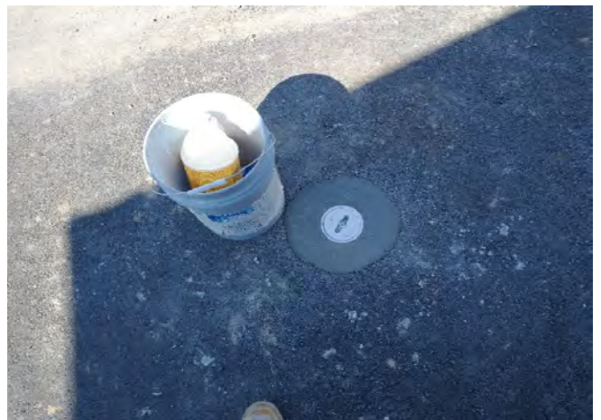
Newly installed buried line cleanout
