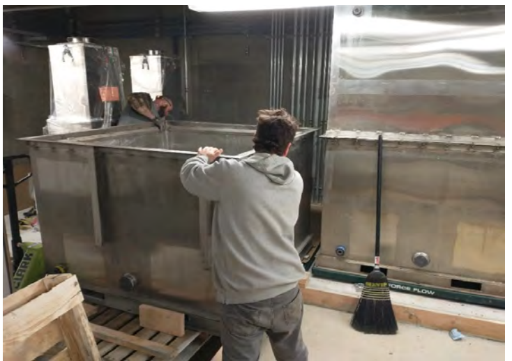
Installing new 1000-gallon batch tanks
