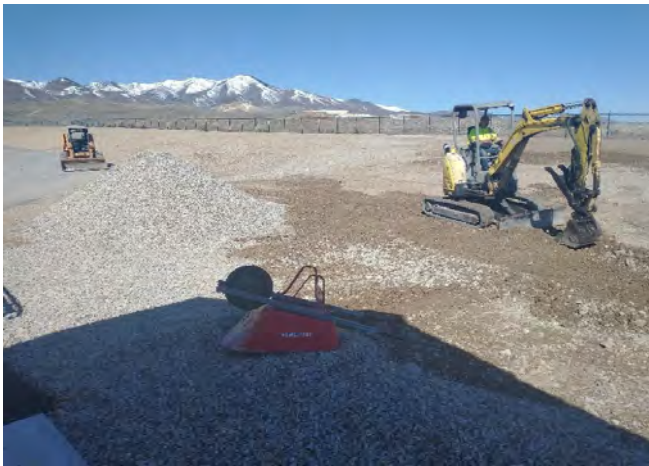
Contractor doing site work to restore proper drainage of property
