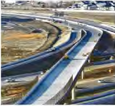
Scott G. Winkler, Deseret News The Farmington section of the West Davis Corridor, which connects western Davis County communities with a viable alternative to I-15, is pictured on Jan. 2.
