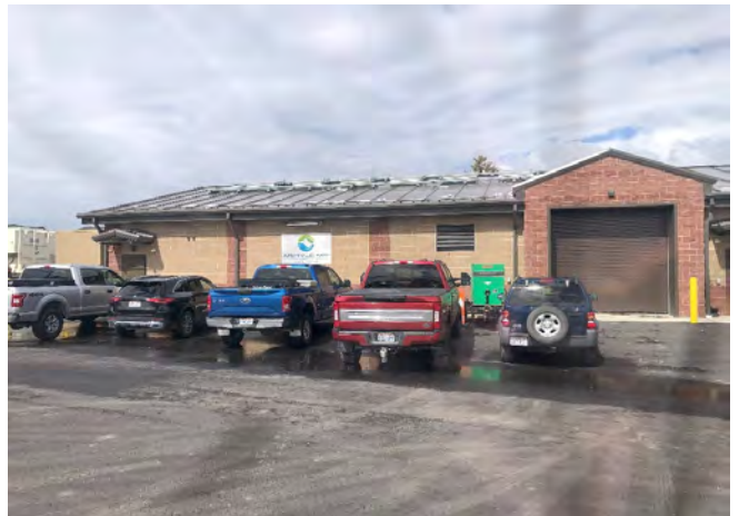
Exterior of the new pumpstation with JVVCD logo installed
